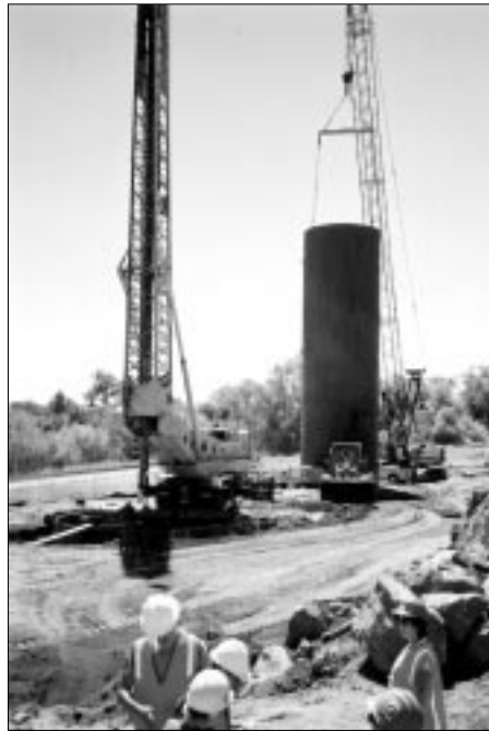
Above: The Geysers Pipeline under construction near The Russian River & Hwy. 101.
